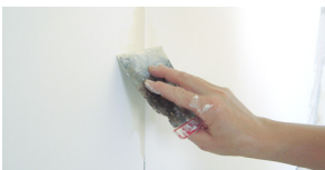
Treatment of the joints
