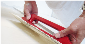
Gluing of the panels
