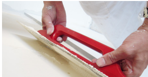
Gluing of the panels
