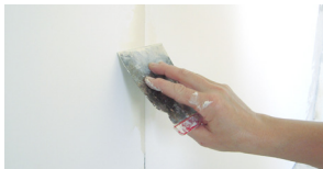
Treatment of the joints
